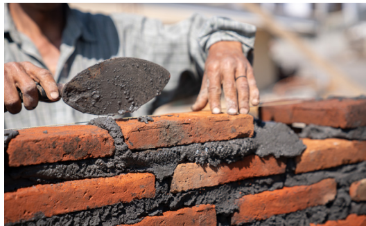
Construction and brickwork
