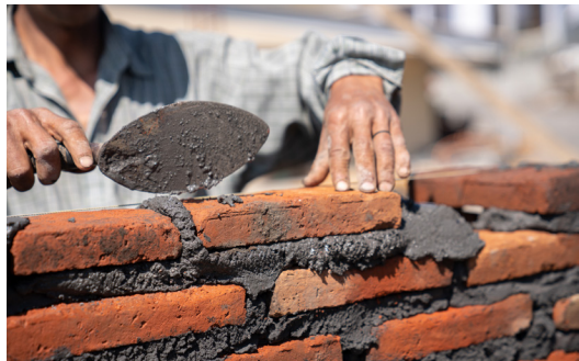
Construction and brickwork
